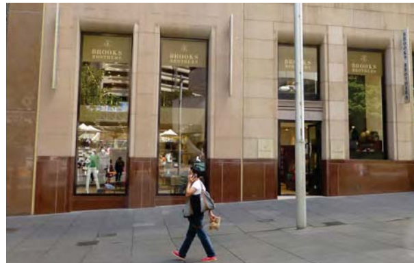
Adapted heritage building. Brooks Brothers, 44 Martin Place
