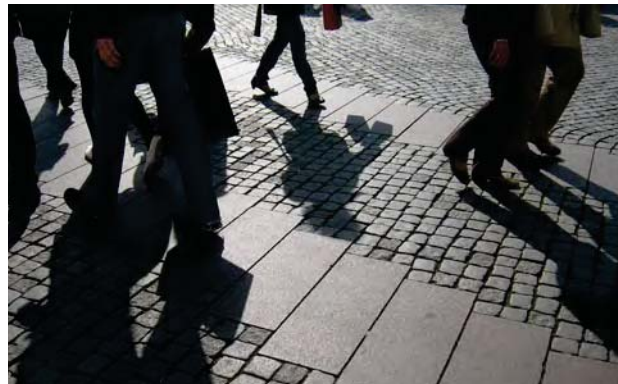
The crossing zone is a mix of different types of pavers, but all of the same material and colour. Malmö, Sweden
